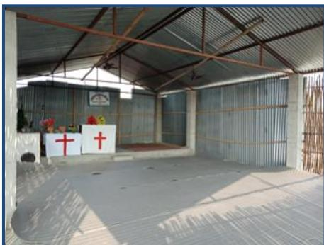
This church has a concrete floor and corrugated iron roof, but its walls are not fully waterproof.
